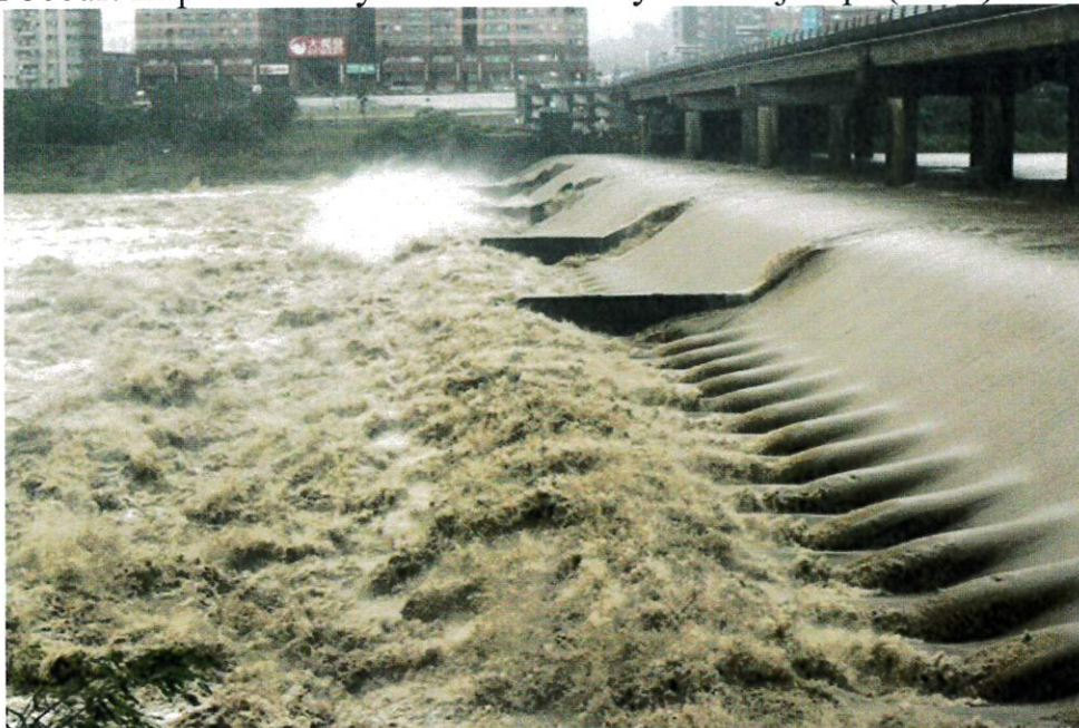
Fig. 2 A photo of hydraulic jump
