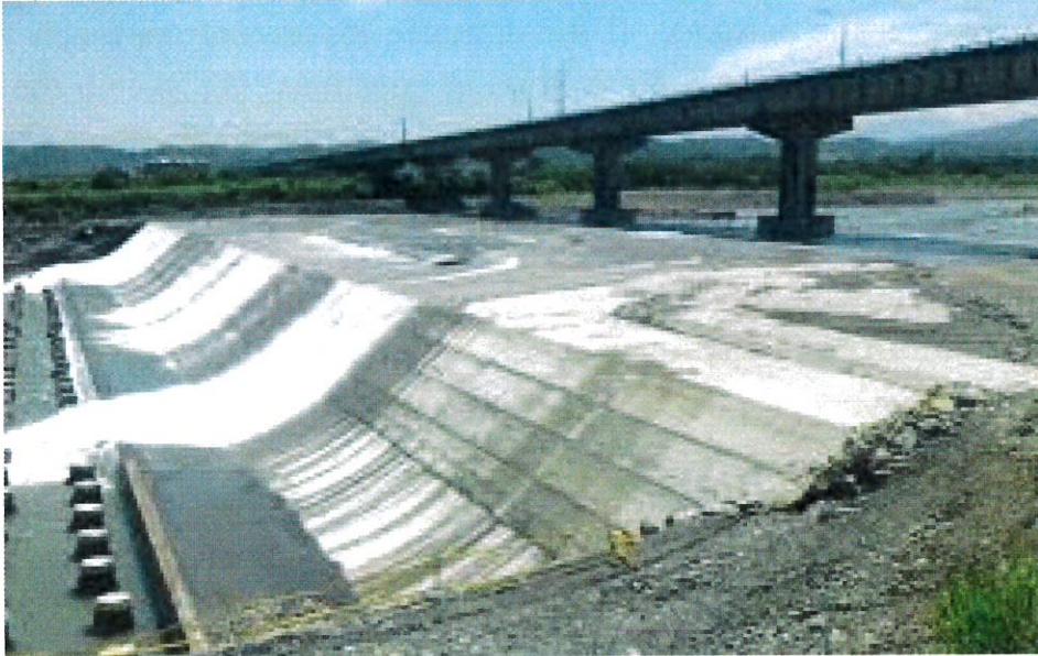
Fig. 1 Drop structures of Zhongzheng Bridge over the Touchien river, Hsinchu
